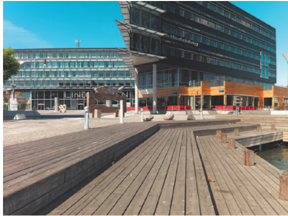
Camera positioned level. The roof of the building is outside the area projected onto the sensor (HC28 + HTS).
